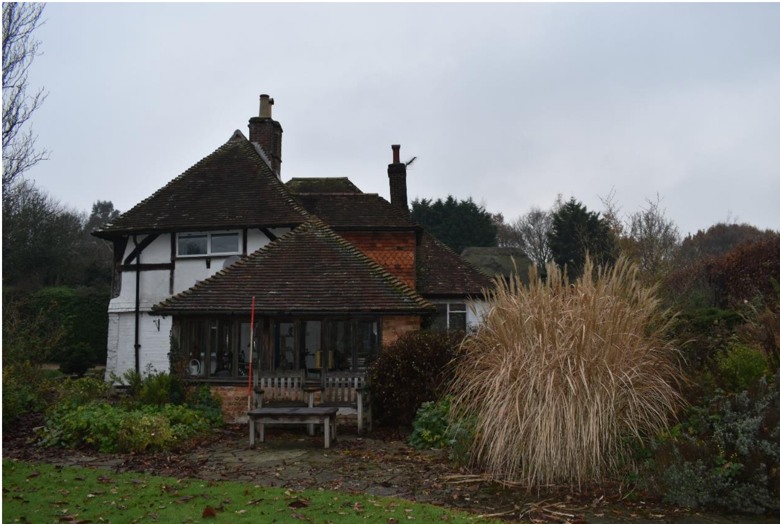
Plate 10: View of south eastern side of Church Hill Cottage (looking north west)
