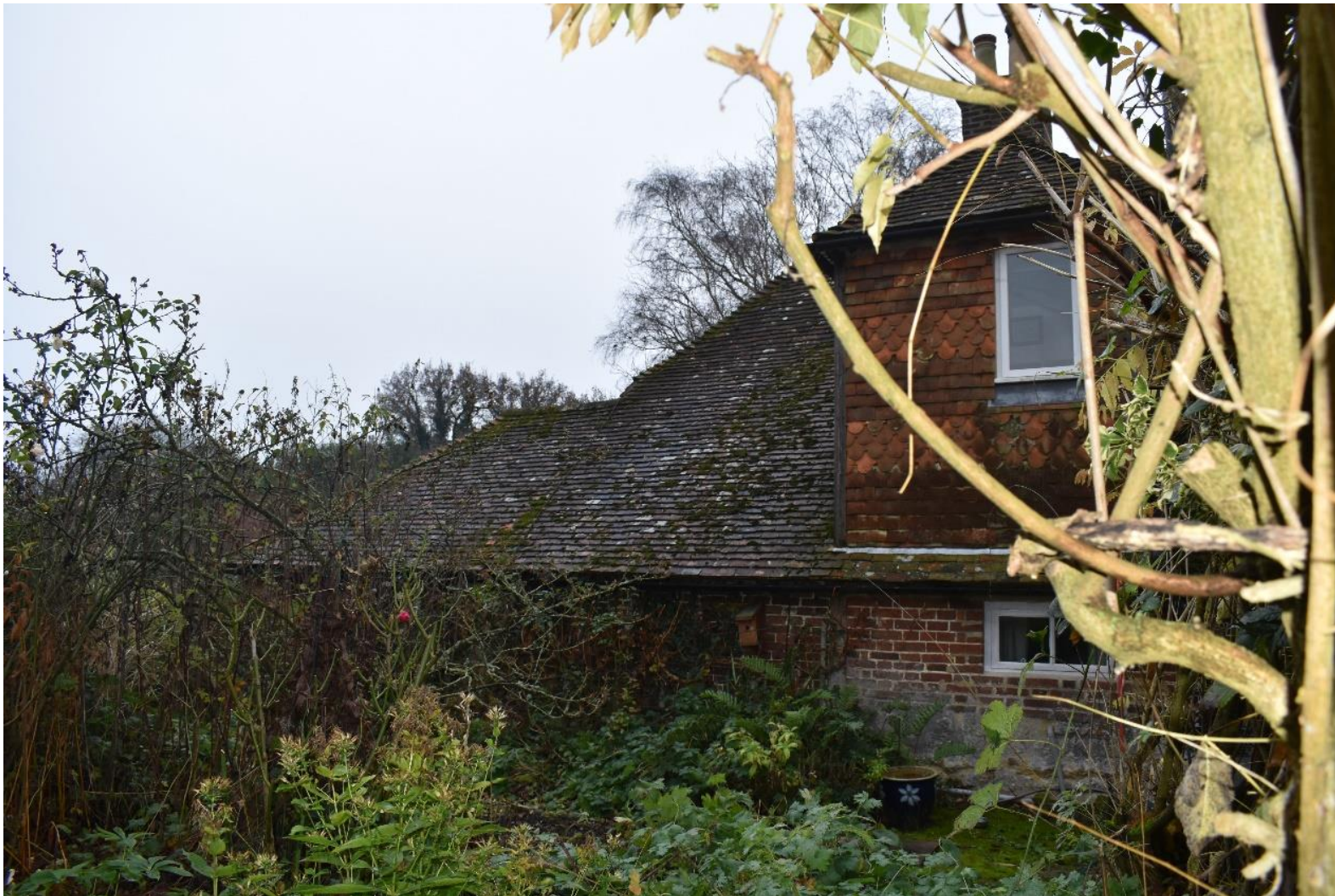
Plate 13: View of part of the rear of Church Hill Cottage (looking south)
