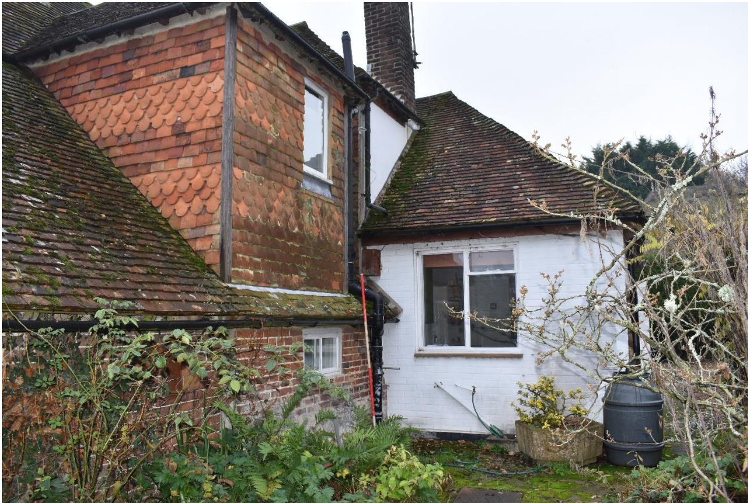
Plate 12: View of part of the rear of Church Hill Cottage (looking west)
